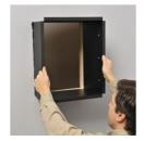
Slide the EasyMount<sup>TM</sup> sleeve through the wall penetration so that the flanged area of the sleeve sits flush with the surface of the wall. Ensure the EasyMount<sup>TM</sup> sleeve is level and plumb prior to fastening to the existing studs.
