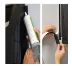
Seal joint between EasyMount<sup>TM</sup> sleeve and Wine Guardian system on the flange side of system with a latex caulk to ensure a tight seal and prevent the system from horizontal movement. After caulking add the kit supplied self adhesive insulate strips tight to the chassis and cover the wall sleeve flanges to prevent possible sweating.
