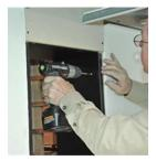
Fasten the EasyMount<sup>TM</sup> sleeve to the wall studs through the six (6) pre-drilled holes located on either side of the EasyMount<sup>TM</sup> sleeve. Start by inserting a wood screw into the lower pre-drilled holes on both sides of the sleeve, and tighten until snug. Do not over tighten. Then insert screws into the upper pre-drilled holes on both sides of the sleeve, continue to middle set of holes. Ensure screws are flush with wall sleeve inside surface. Do not over tighten.
